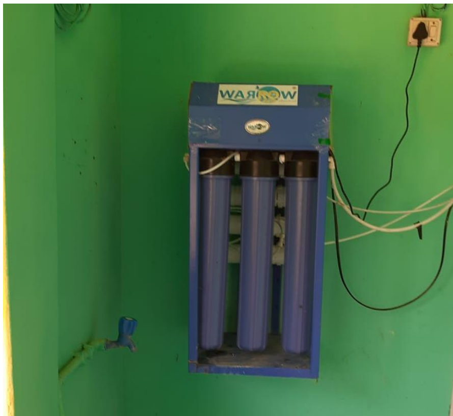
DRINKING FACILITIES FOR NON-TEACHING STAFF
