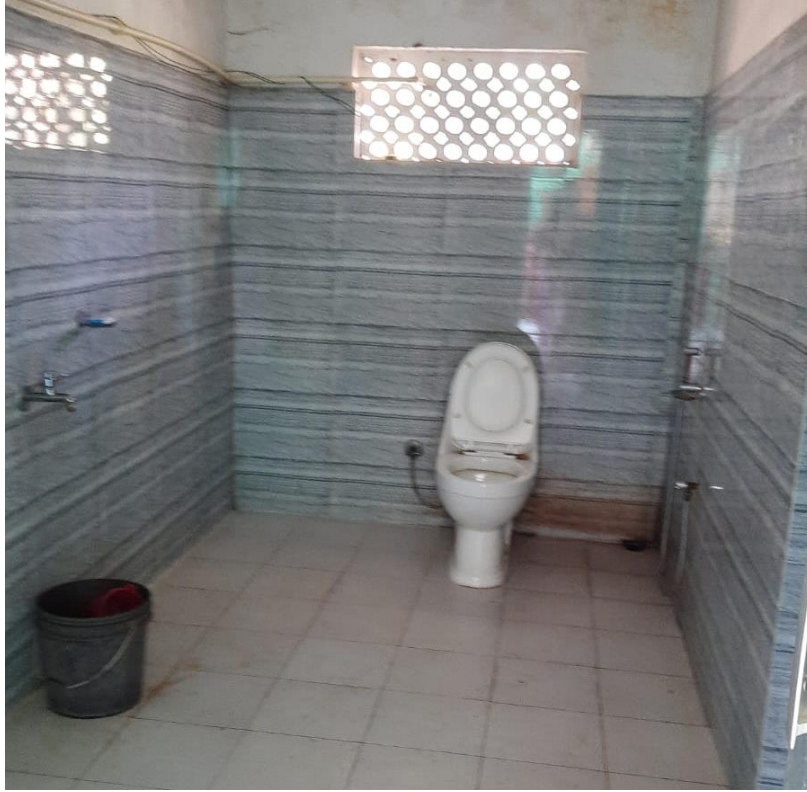
WASHROOM FACILITIES FOR NON-TEACHING STAFF
